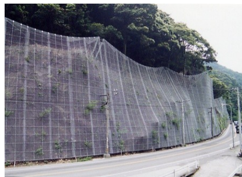
Figure 1. Falling rock protection net
