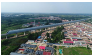
Figure 1. Sound barrier accurate picture
