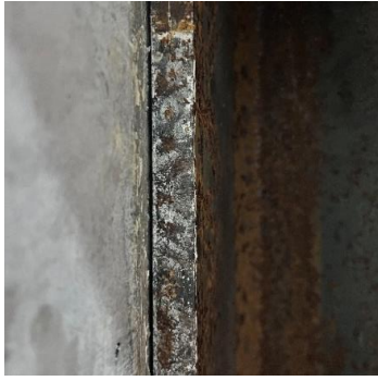
(e) P-C-16-40-10 separation of steel beams and concrete
