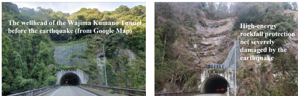
Figure 15. The wellhead of the Wajima Kumano Tunnel
