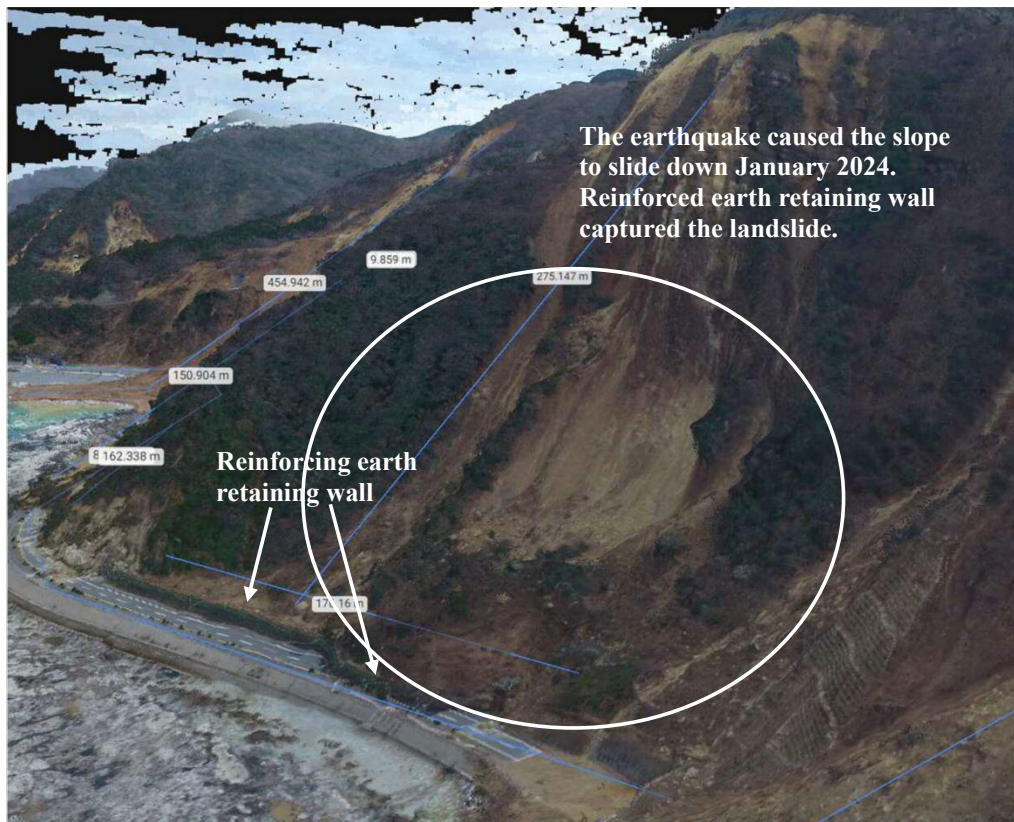
Figure 13. Suzu Maura (Sediment capture by reinforced soil retaining wall)
