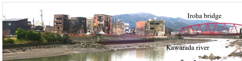
Figure 9. Morning Market Street ( Wajima ) where the fire occurred
