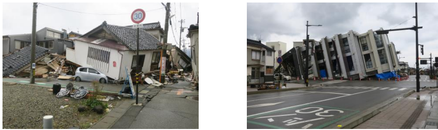
Figure 8. House and building in Wajima that collapsed due to the earthquake
